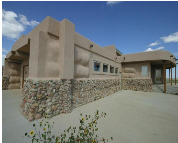
Figure 6 – Southwest View of Tire Bale House near Fountain, Colorado
